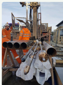
Preparing a memory tool string on site
